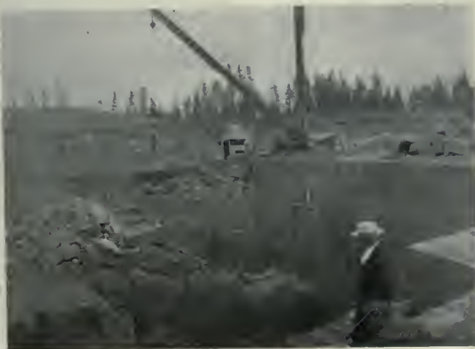
Sackville Sandstone Quarry, Sackville, N.S.
